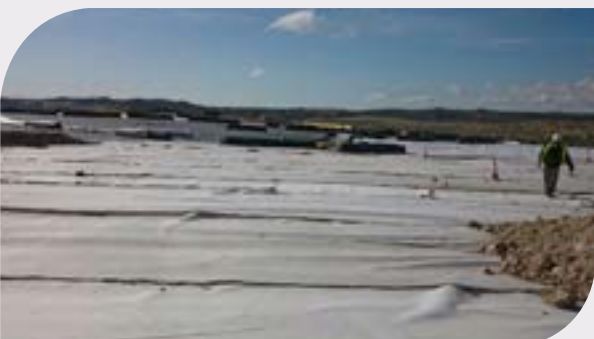
Valmadrid Landfill (Spain) – 433.000 m 2 CAPDRAIN
