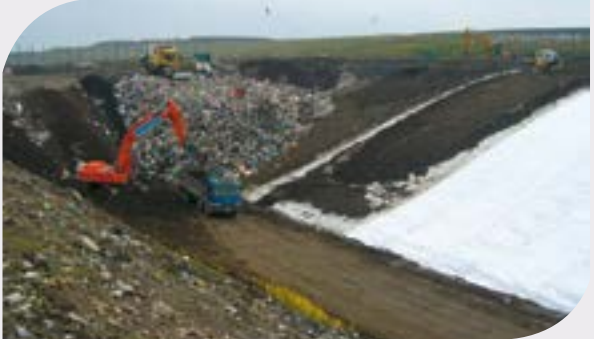
Ballealy Landfill (Ireland) – 200.000 m 2 TECHDRAIN
