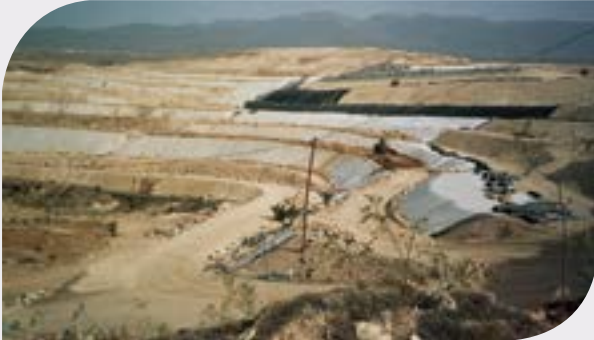
Indaver Landfill (Belgium) – 40.000 m 2 TECHDRAIN
