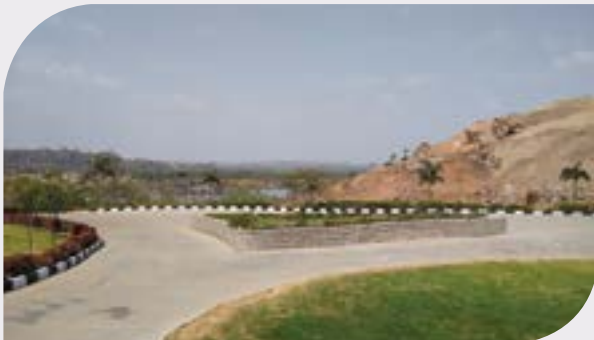
Hyderabad Landfill (India) – 550.000 m 2 CAPDRAIN
